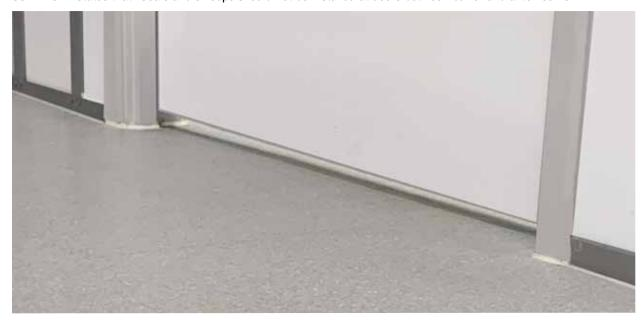
Figure 2: Caulked Modular Walls and Ceiling
